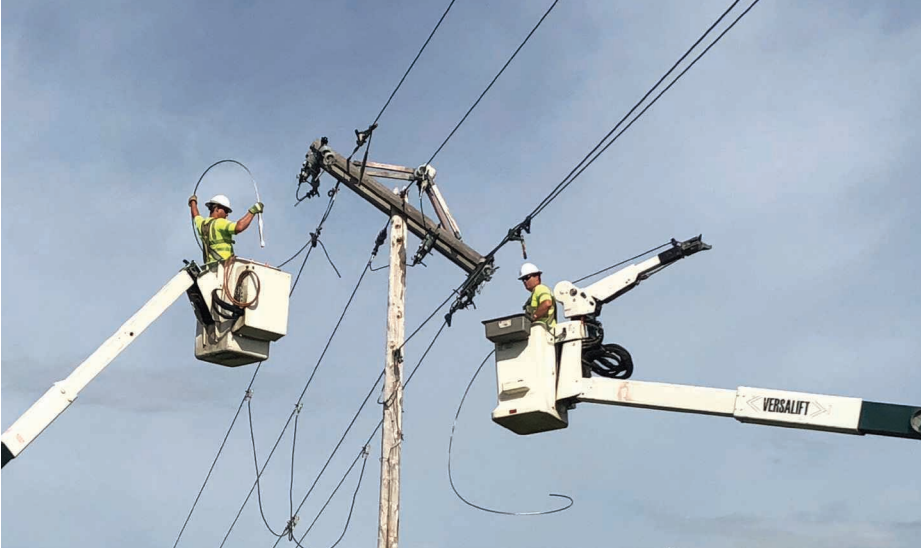
Renville-Sibley linemen, thank you for keeping the lights on! Here our linemen are repairing a broken structure. 405000
