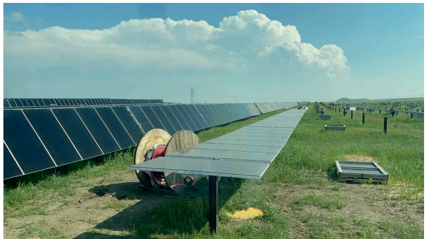
A look on the ground as crews prepare the Wild Springs Solar Project for power generation. Photo submitted by East River Electric
